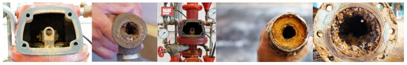
This testing is required by NFPA 25 (National Fire Protection Association) Standard for Inspections, Testing and Maintenance of Water-Based Fire Protection Systems in Chapter 14
